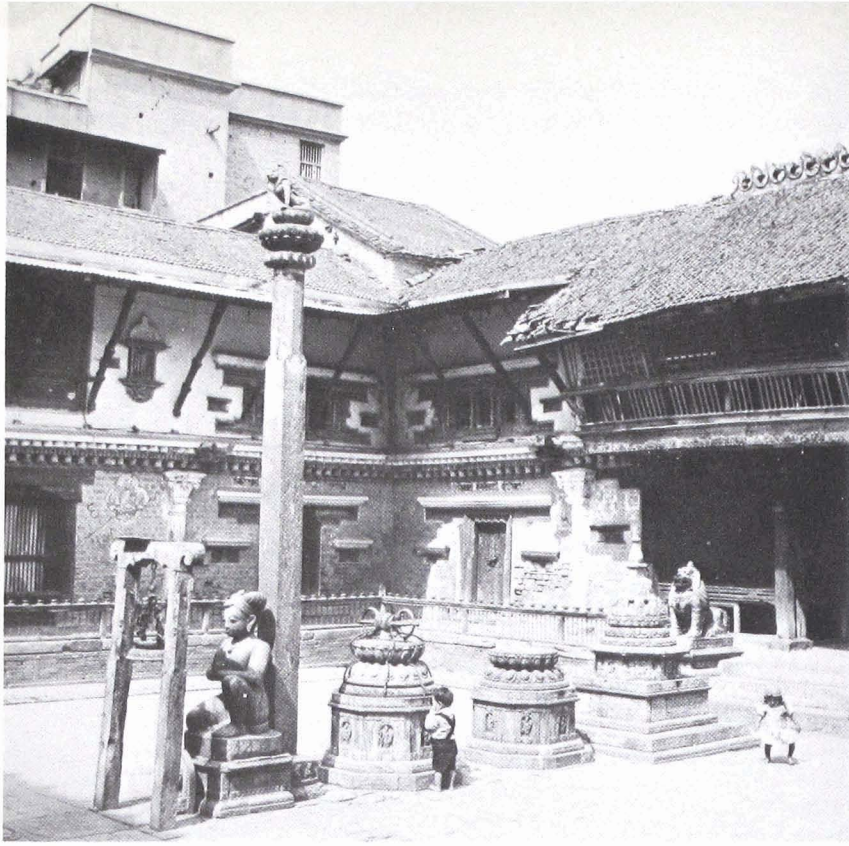
55. Inner courtyard of Oku Bāhāl, Patan.
